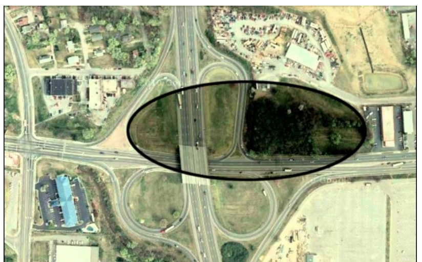
Footprint of Old Lick Cemetery before construction of the 581-Orange Avenue interchange.
