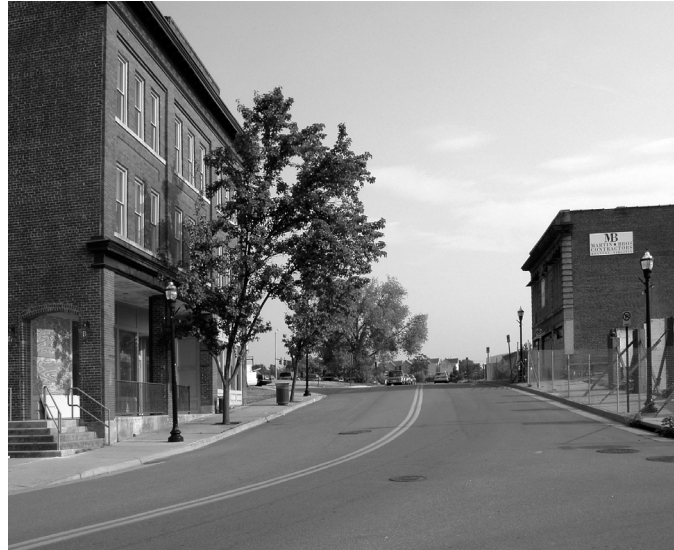
Looking north on Henry Street: The three-story, 70,000 square-foot Social Security building would go in the next block, behind the building on the left. Henry Street would be closed to traffic at that block.
