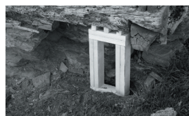
Clockwise from above: The meathouse at the end of the day. The meathouse earlier that morning. Ruth Doan mixes a borate solution before applying it to the logs. Doubled 2-by-4 lumber helps support a corner where a deteriorated log has been removed.
