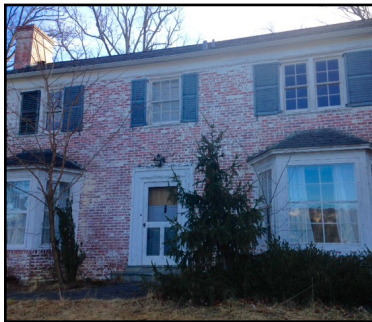
Wood's End House (Prior to 2015 demolition)
