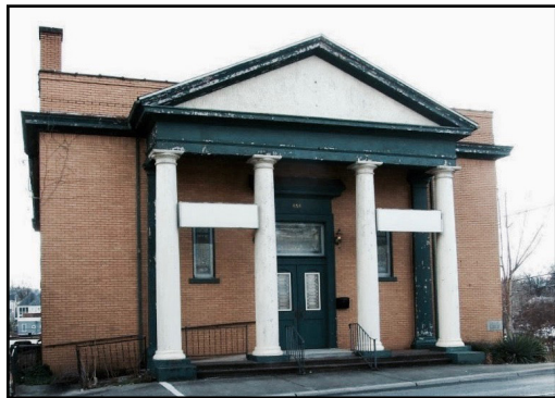
Christian Science Church pre-renovation
