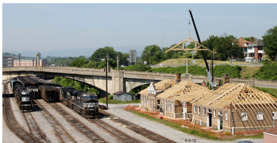
Progress as of early May on Phase I of the Virginian Railway station restoration.
