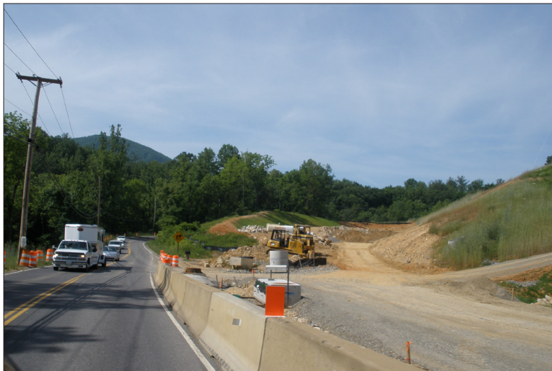
The addition of two lanes will increase the accessibility of Back Creek and Poages Mill.
