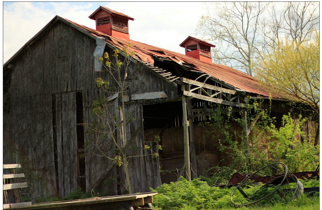
Current condition of the barn at Waskey's Mill.
