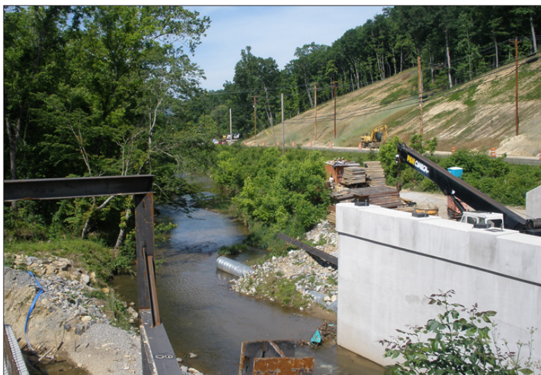
Construction along and over Back Creek.
