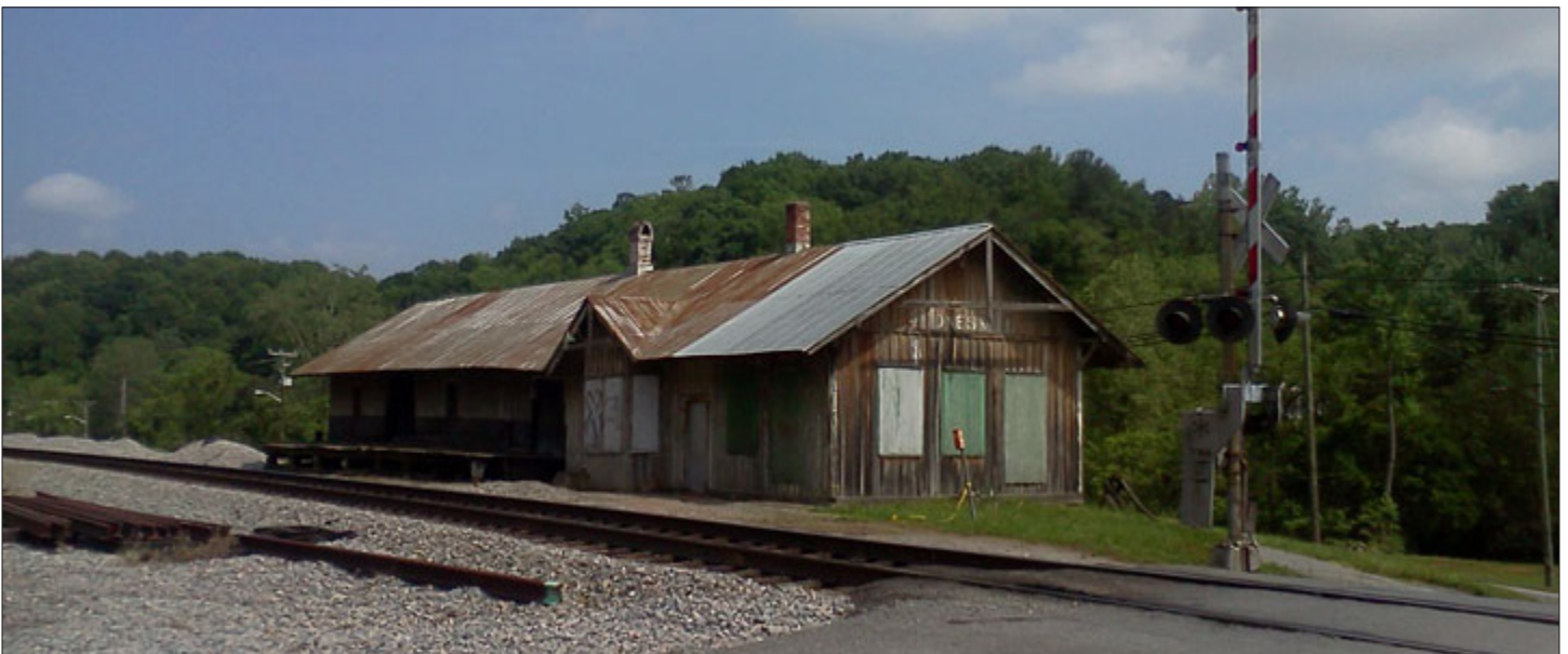
Current condition of the Boones Mill Train Depot.
