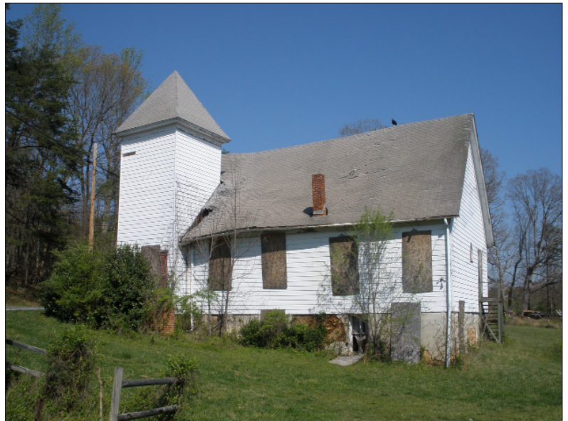
Current condition of St. John's AME.
