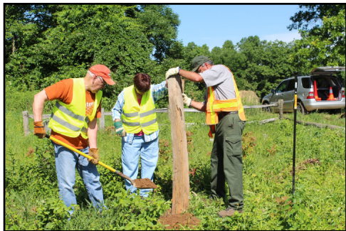
Fence Post Installation at Parkway Cemetery
