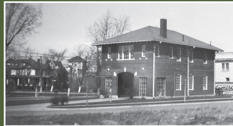
Photograph ca. 1922, looking northwest (Virginia Room, Main Library, Roanoke, VA)
