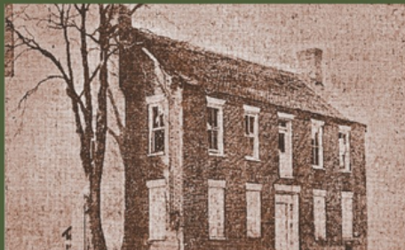
The ca. 1825 William Persinger House from the 1959 Roanoke Times & World News article written by Raymond P. Barnes. Note the vacant condition of the house. The house overlooked the Roanoke River. It was demolished in 1963 for an industrial office complex.
