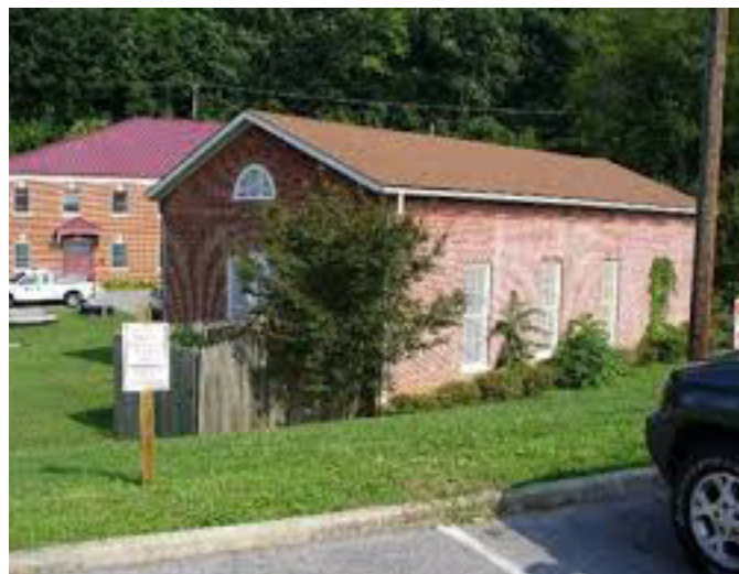
Exterior of Crystal Spring Pumping Station
